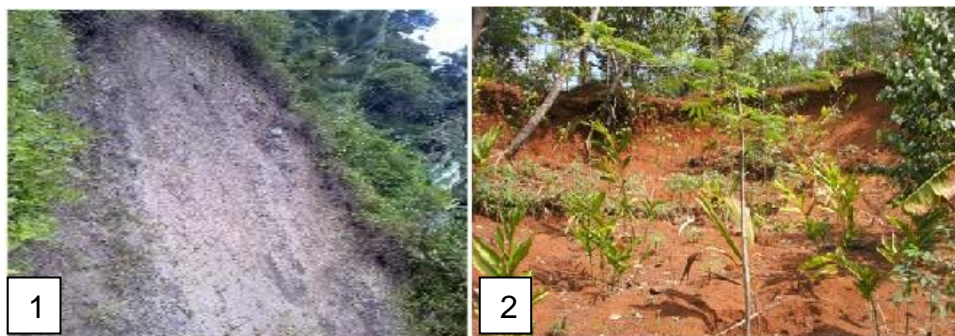
Figure 9. Landslide Appearance Photos in 1. Krajan Village, 2. Village Semedo, (Source: Suwarno, 2014)
