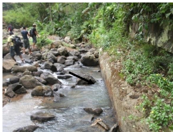
Figure 4. The appearance of a fault (Source: Suwarno, 2014).
